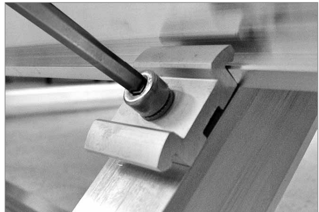
Tightening the lower clamps
