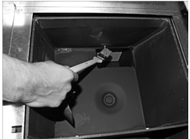
Abb. 29: Thermocontrol-Sensor reinigen
